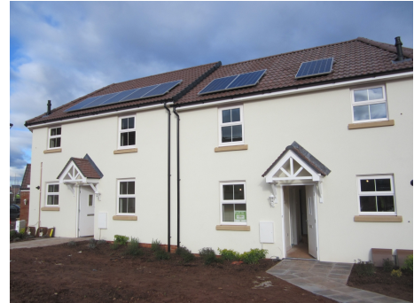
Picture 12 Photo-voltaic roof panels
